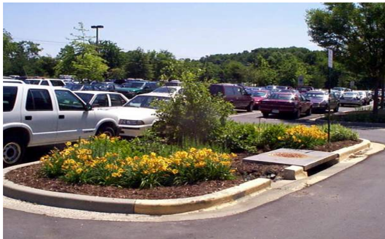
Photograph WQ-13 – Example of a Porous Detention Island. This porous detention island is designed to reduce runoff rates and volumes and pollutant loading.
