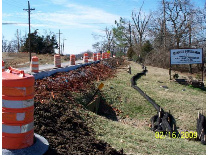
Photograph CS-7 – Example of Fiber Roll/Wattle
