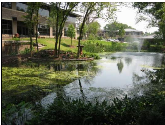
Photograph WQ-2 – Example of an Extended Wet Detention Basin.
