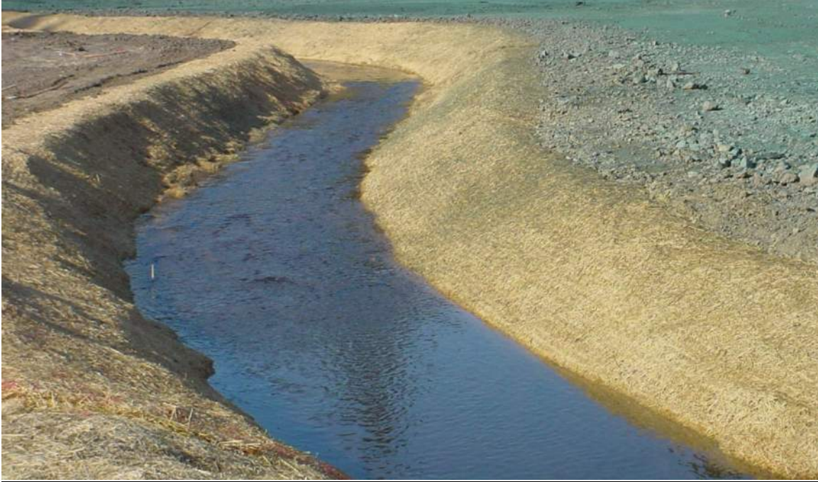
Photograph CS-3 – Example of Erosion Control Blanket
