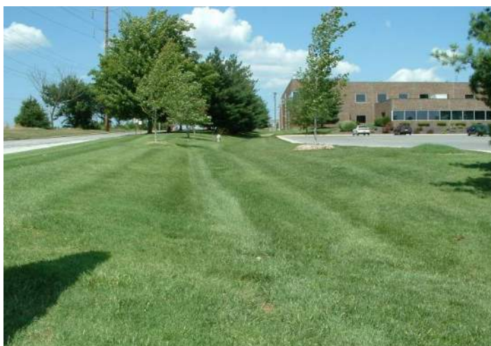
Photograph WQ-8 – Example of a Grass Buffer.
