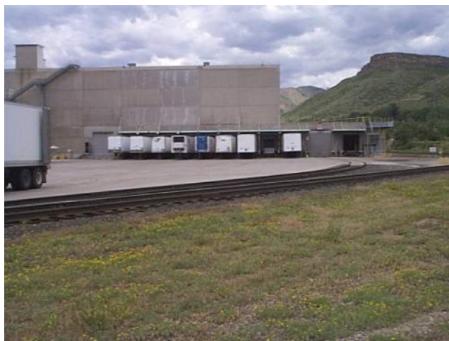
Photograph WQ-10 – Example of Covered Storage/Handling Area.
