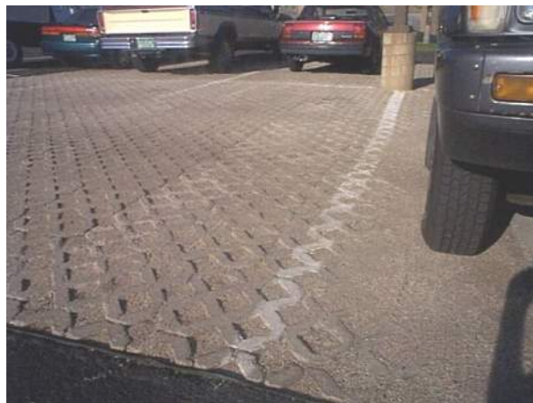
Photograph WQ-6 – Example of Modular Block Porous Pavement.
