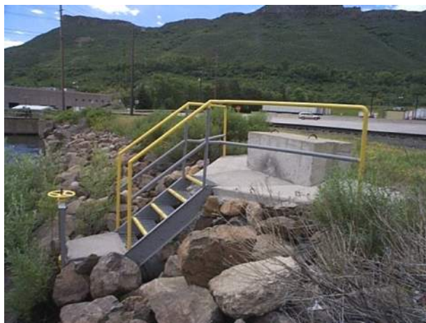
Photograph WQ-11 – Spill containment structure with valve control.
